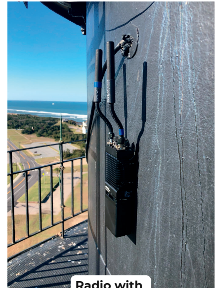
Radio with MAGNETIC MOUNT PLATE on an iron lighthouse.
